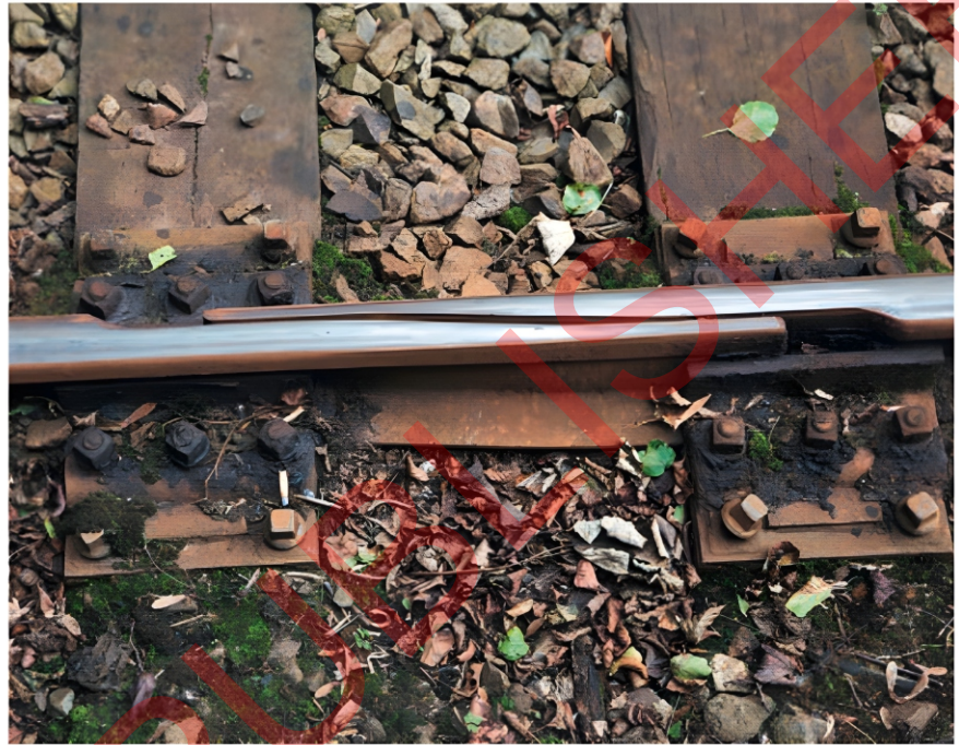
Figure 1.9: Tapered rail overlap to accommodate thermal expansion.
