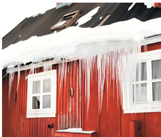
Figure 1.7: Snow patterns on a roof reveal areas of heat conduction and insulation.
