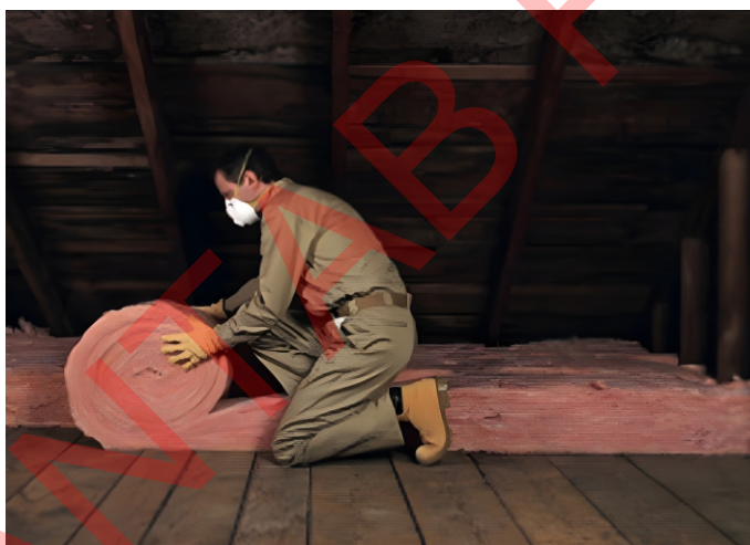
Figure 1.21 (a). Installing thermal insulation to reduce heat loss through the roof.
