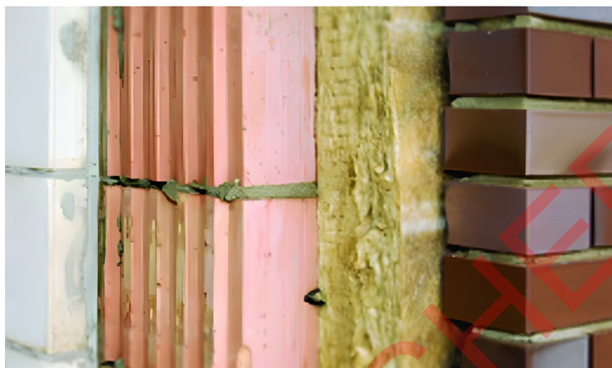
Figure 1.21 (c): Cavity wall insulation reduces heat loss.
